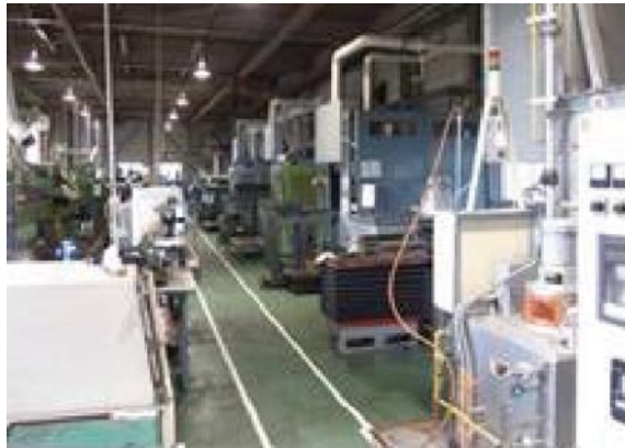
Figure 38 Heat treatment line
